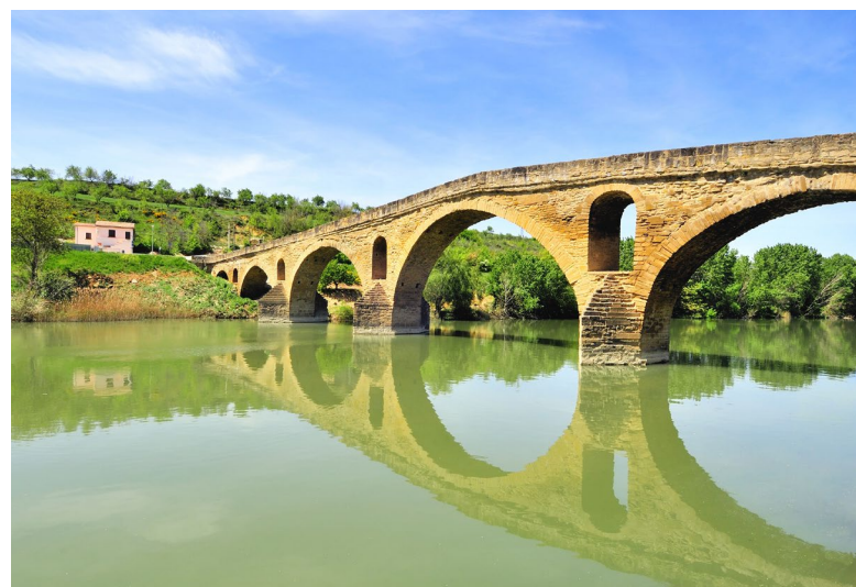
▼ LA REINA BRIDGE NAVARRE
